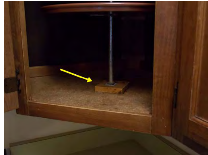
Older cabinets required an additional shim to improve support for the rotating tray (Lazy Susan).
