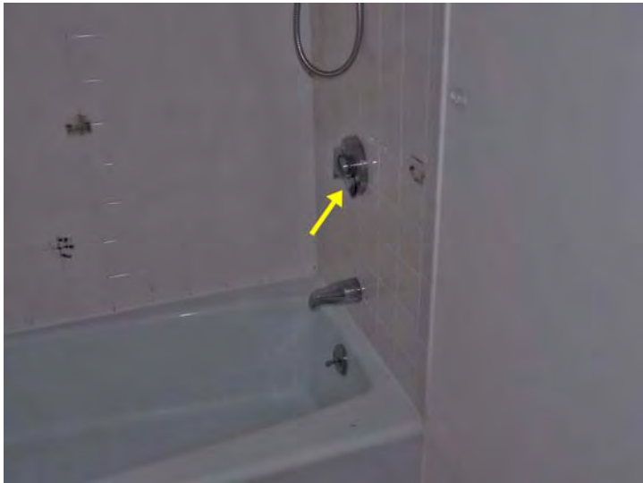
Bathtubs/showers have an anti-scald mixing valve.
