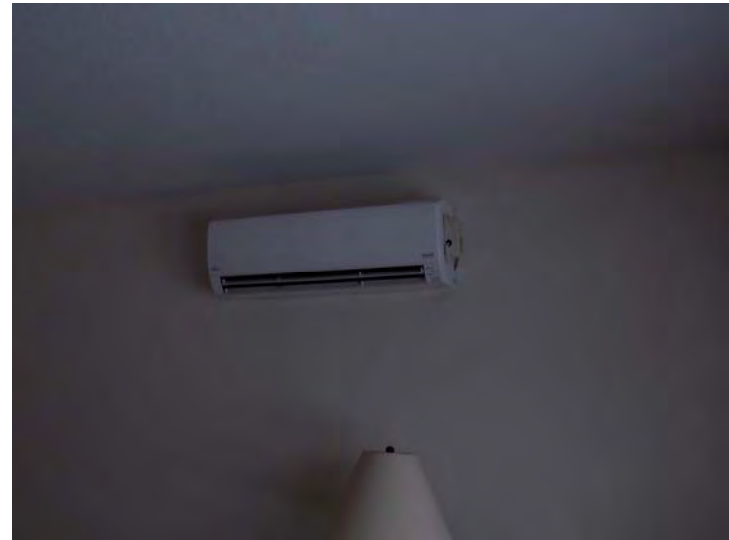
A view of one of the heat pump terminal units.
