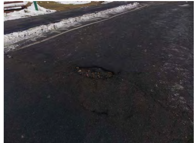
A close-up of a damaged section in the main parking lot.
