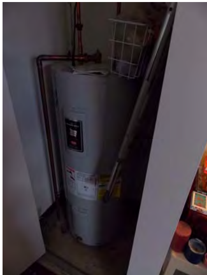
Every apartment has an electric-heated DHW tank.
